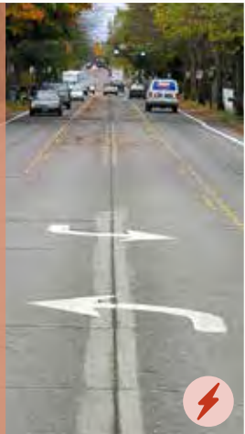
ROADWAY DIET OR CLOSURE | DIETA O CIERRE DE CARRETERA
