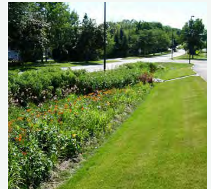
Bioswales are linear stormwater management systems that infiltrate, slow, and clean water when it rains
