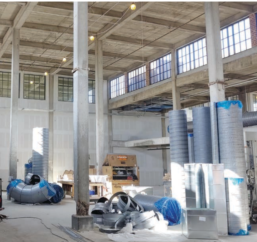
Interior shell space with demising walls and clerestory windows
