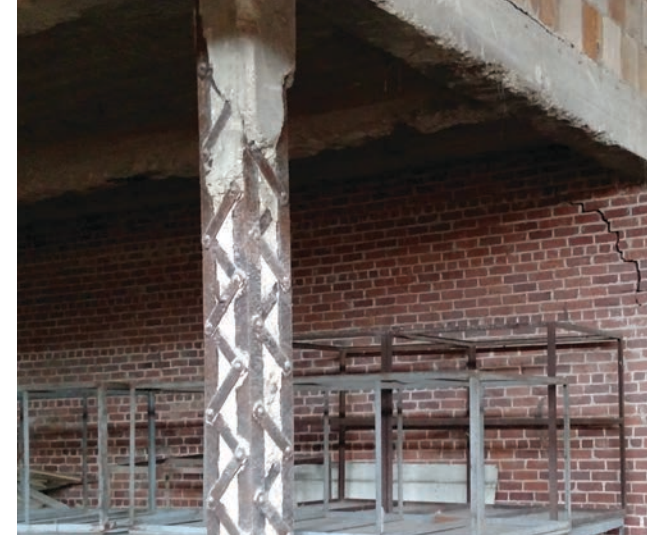
Structural damage to columns and brick walls
