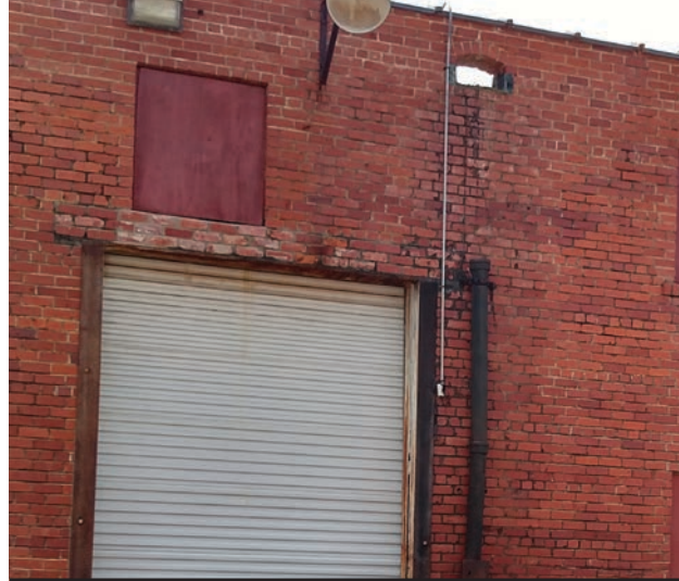
Missing brick, windows, & unoriginal openings
