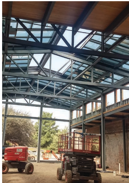
New roof structure including retractable glass
