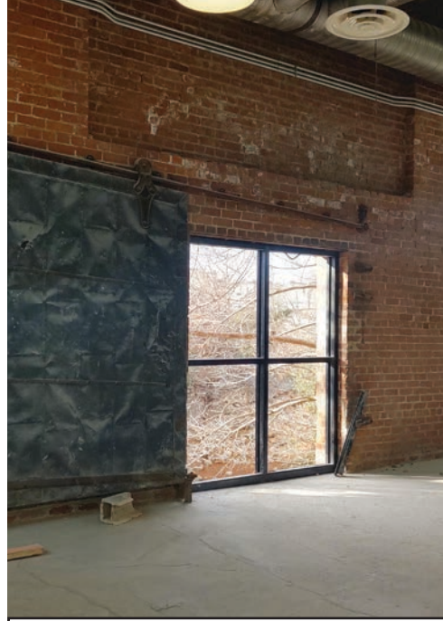
Preservation of original historic fire doors
