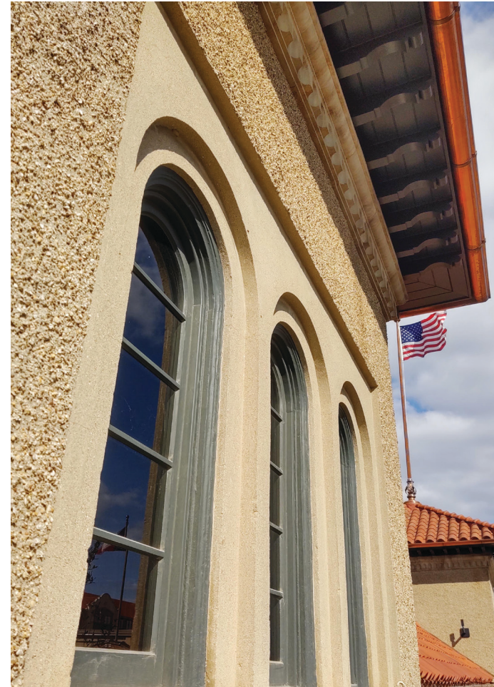
Fully restored windows, tower roof, and flagpoles
