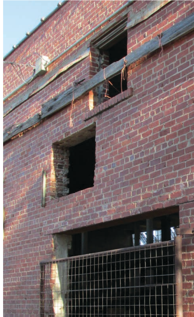
Missing brick, windows, & unoriginal openings
