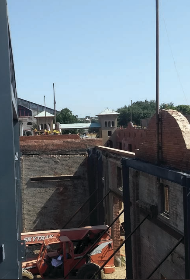
Addition of new Barn F roof where existing roof was damaged by 1940s fire. The new roof was designed to mimic the original clerestory footprint
